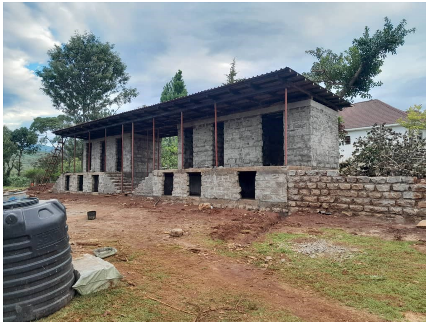
Baufortschritt Kshek Vocational Skill Centers
