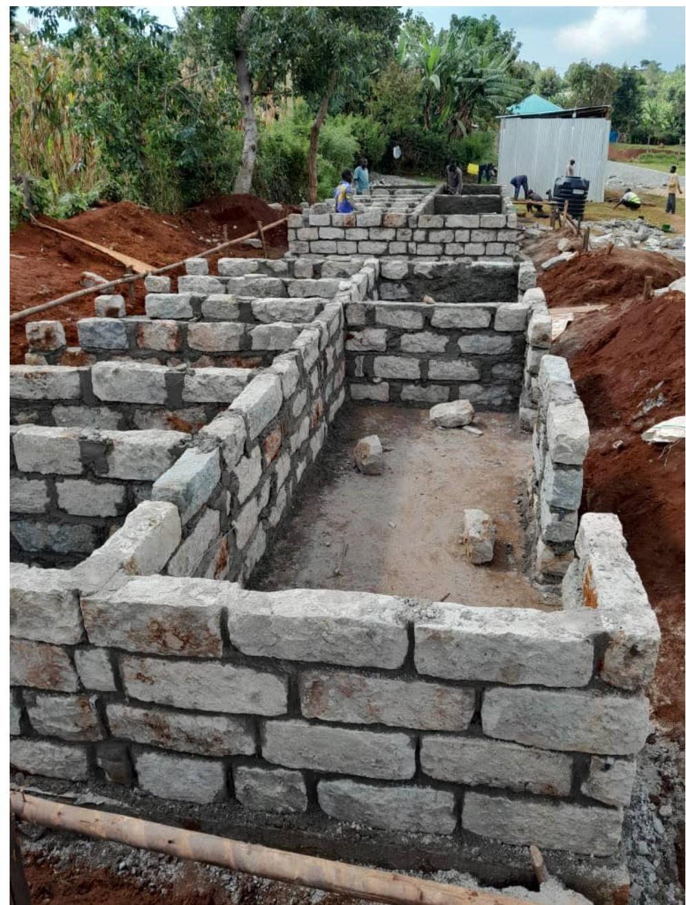
Baufortschritt Kshek Vocational Skill Centers
